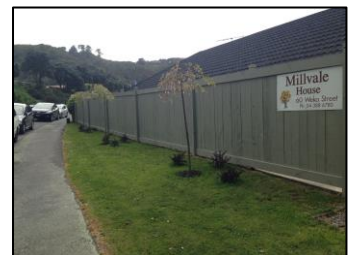
Our beautiful new perimeter fence and signboard
